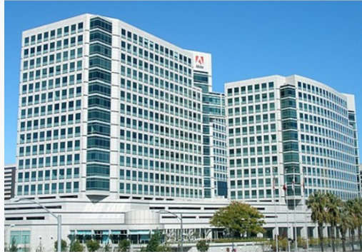
Adobe World Headquarters in San Jose, California
