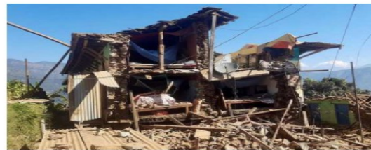
Badly hit: Houses damaged in the aftermath of an earthquake at Jajarkot of Nepal, on Saturday. AP
