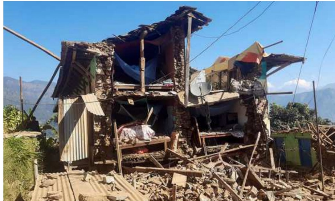
Badly hit: Houses damaged in the aftermath of an earthquake at Jajarkot of Nepal, on Saturday. AFP
