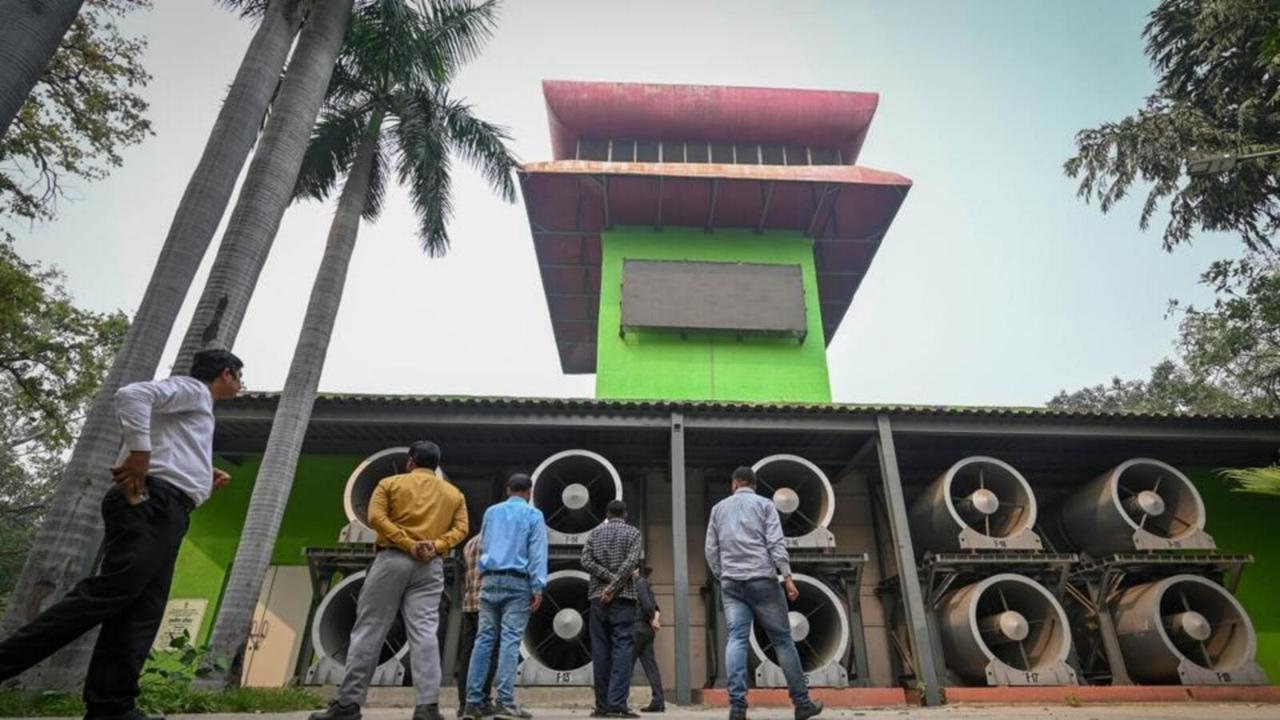
1. C) 50%. The smog tower at Connaught Place, New Delhi, has been found to clean air with 50% efficiency, but this efficiency drops to 30% at a distance of 50 meters from the filters and just above 10% when 500 meters away.
