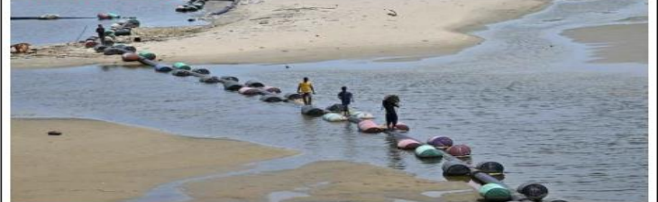
Action plan: Workers clearing the Adyar river mouth in Chennai on Tuesday. The Water Resources Department has engaged more machinery to clear silt and complete the project by June-end. S. VELAYUTHAN/RJ
