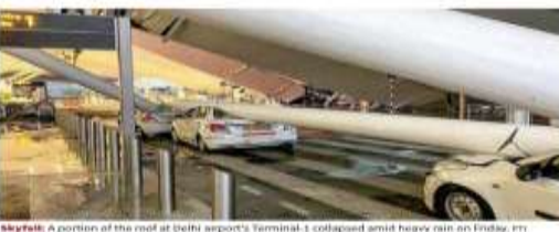
Sanghvi: A portion of the roof at Delhi airport's Terminal-1 collapsed amid heavy rain on Friday. PTI
