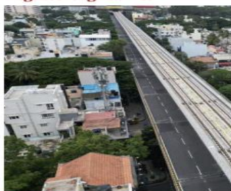
Two-in-one: Bengaluru Metro Rail Corporation Ltd. will soon inaugurate South India's first road-Metro flyover, which starts at the Ragi Gudda Metro station and ends at the Silk Board junction. The 2+2-lane flyover gives a smooth ride with three U-turns. K. MURALI KUMAR
