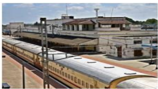
The Railways will soon dispense with the method of stationmasters setting time on the instructions of section controllers.
