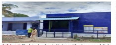
Safety net: The fair price shop in Masinagudi has been remodelled with a three-tier security system. SPECIAL ARRANGEMENT
