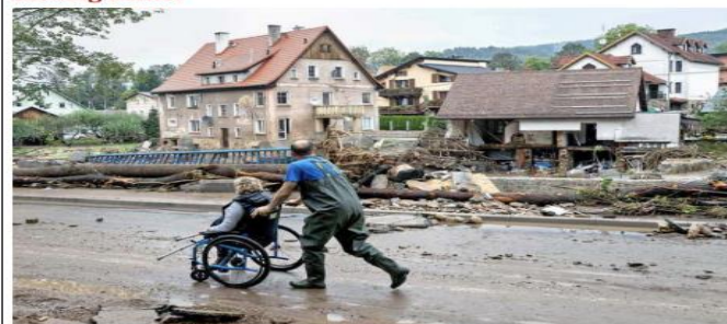
A resident pushes a woman in a wheelchair past a destroyed building following the floods in Ladek-Zdrój, southern Poland, on Monday. Flooding sparked by Storm Boris in central Europe has burst dams, knocked out power and killed at least 17 persons. AFP
