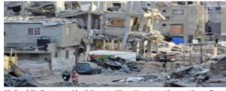
Major hits: Destroyed buildings in Khan Younis in the southern Gaza Strip after the ongoing war between Israel and Hamas. AFP
