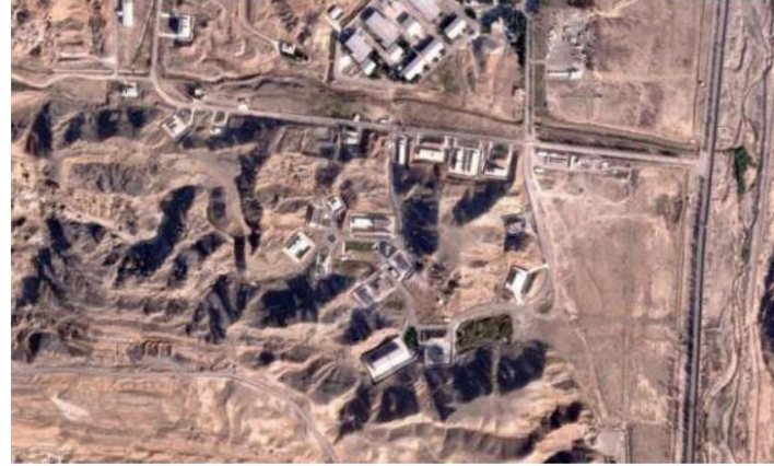
Hit hard: Satellite image shows damaged buildings at Iran's Parchin military base on Sunday. AP
