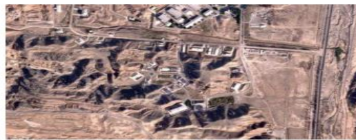
Hit hard: Satellite image shows damaged buildings at Iran's Parchin military base on Sunday. AP
