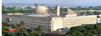
Punjab and Haryana share the Vidhan Sabha complex, designed and built by French architect Le Corbusier, in Chandigarh. FILE PHOTO
