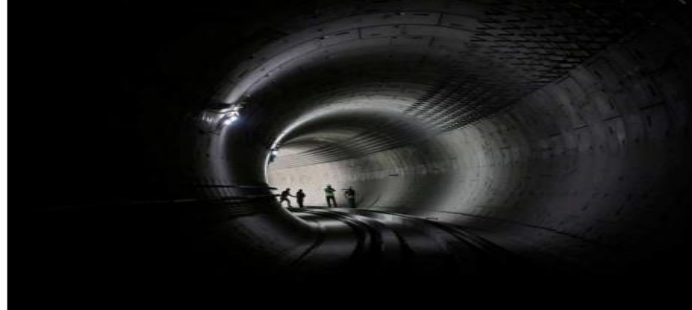
Subterranean transit: Workers in a tunnel built for the Mahatma Gandhi Road Metro station that is coming up on the Pink Line of the Bengaluru Metro network on Monday. The station will be an interchange transit point between the pink and purple lines. FILE PHOTO K.
