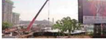
The hoarding in Chhatrapati collapsed on May 13, 2024
