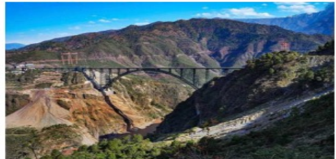
Blazing heights A view of the 'world's highest railway bridge', built at a height of 359 metres over the Chenab river in Jammu and Kashmir's Reasi district, which witnessed the maiden run of a track-mounted trolley on Sunday. The ₹1,496-crore Chenab railway bridge is part of the Udhampur-Srinagar-Baramulla Rail Link project, which will connect the Kashmir Valley with the rest of the country. PTI REPORT ON PAGE 18
