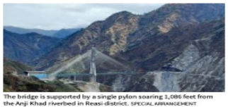
The bridge is supported by a single pylon soaring 1,086 feet from the Anji Khad riverbed in Reari district. SPECIAL ARRANGEMENT
