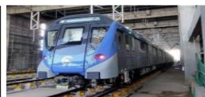
On track: One of the challenges is to complete the laying of the track between Poonamallee and Porur as the earliest so that the testing can begin in three months. (AI Photo)
