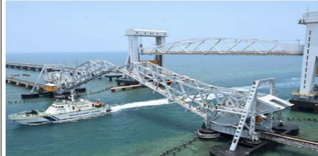
A Coast Guard vessel passes through Pamban channel as Railway authorities filed the vertical span of the New Pamban Rail Bridge during a visit on Wednesday. The Bridge, seen alongside the old one, is likely to be inaugurated by PM Narendra Modi on April 6. BALACHANDRAN
