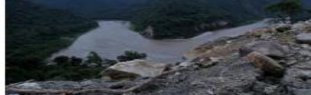
Expensive work: The additional costs of restoring the dam is estimated to be ₹4,189 crore. NLS MWFO
