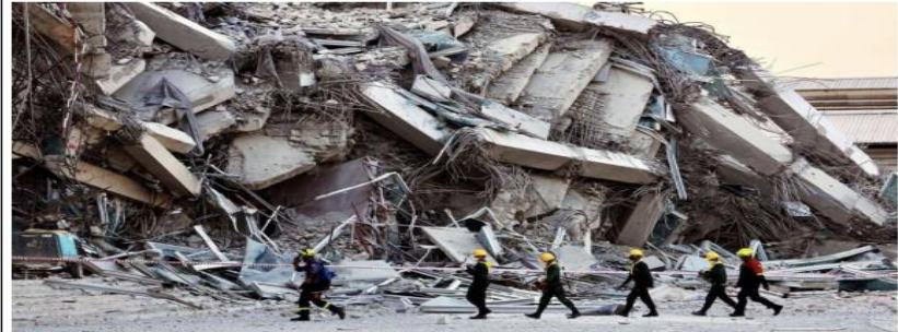
Shells shocked: Rescue workers near an under-construction building that collapsed after the tremor hit Bangkok, Thailand, on Friday.
