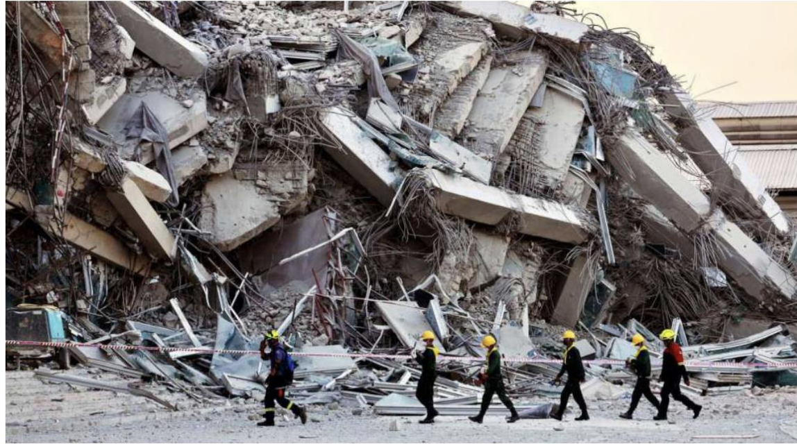
Shell-shocked: Rescue workers near an under-construction building that collapsed after the tremor hit Bangkok, Thailand, on Friday. AP
