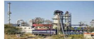
The waste disposal facility at Pithampur where waste from Bhopal's Union Carbide factory has been brought for disposal.
