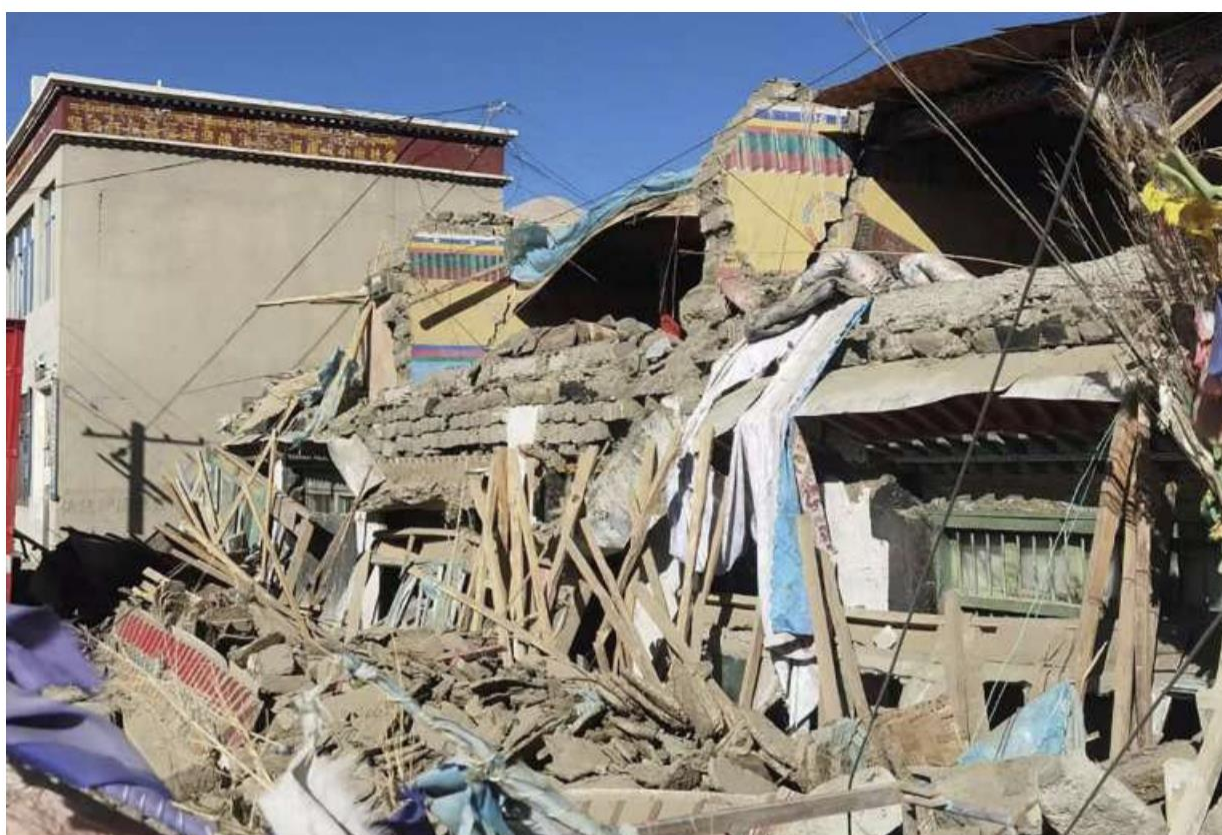
Rubble remains: Damaged houses in Xigaze, Tibet, after the earthquake hit the area. AFP
