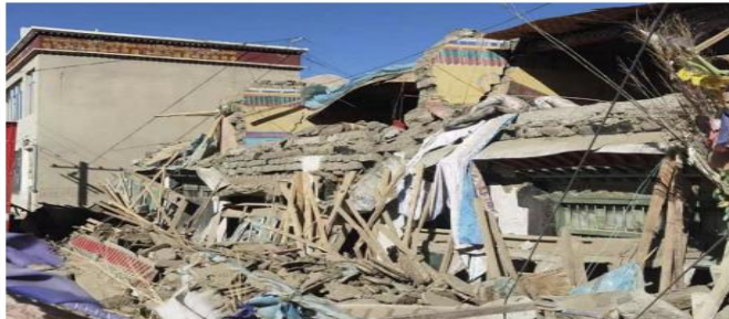
Bubble remains: Damaged houses in Xigaze, Tibet, after the earthquake hit the area. AFP
