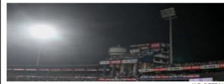
Play in the second India-England ODI in the over-six-decade-old Barabati Stadium was stopped as one of the six towers of the floodlights malfunctioned. The incident happened when the tower adjacent to the iconic clock tower malfunctioned, resulting in a brief stoppage at 6.15 p.m. The lights were restored at 6.45 p.m.
